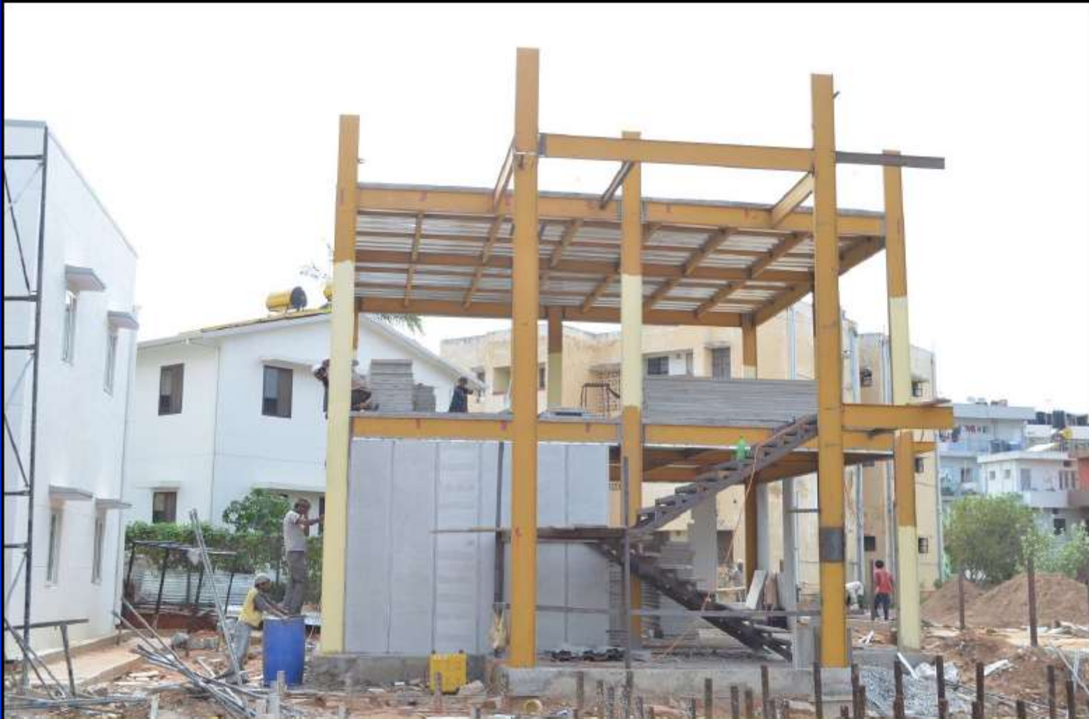
Steel skeleton with Aerocon panel infills
