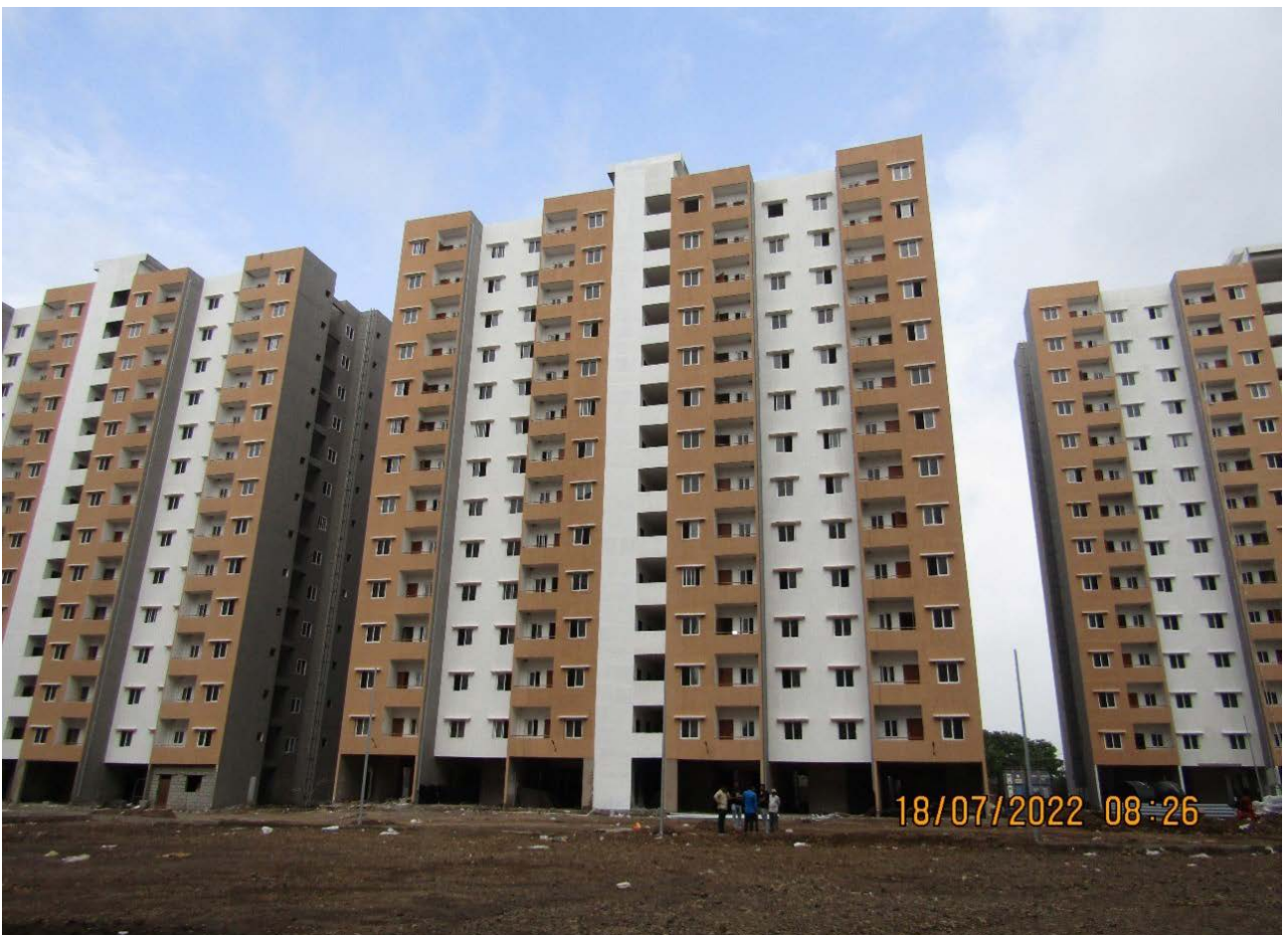
Light House Project at Rajkot under PMAY (U)
