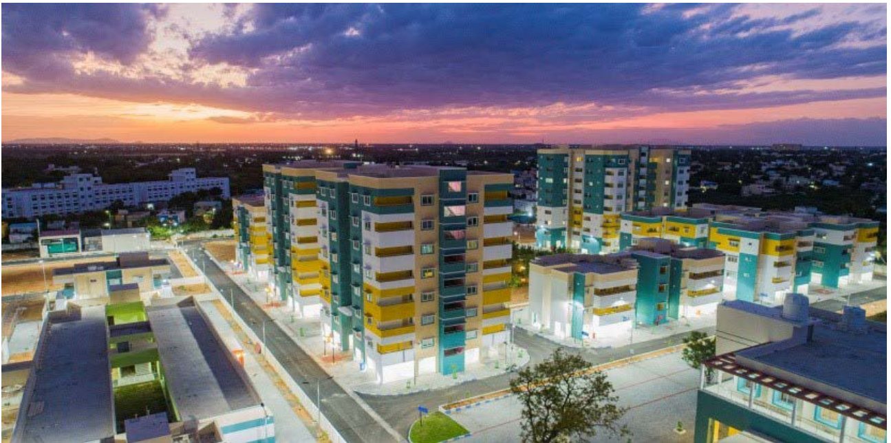
Staff Quarters, Type B (S+7 & S+4), Type C (S+8), Type E (S+2), Hostel Accommodation (S+2), Amenities Block, Security Hut, CSIF Barracks, Dog Kennel & Community Hall at Trichy International Airport
