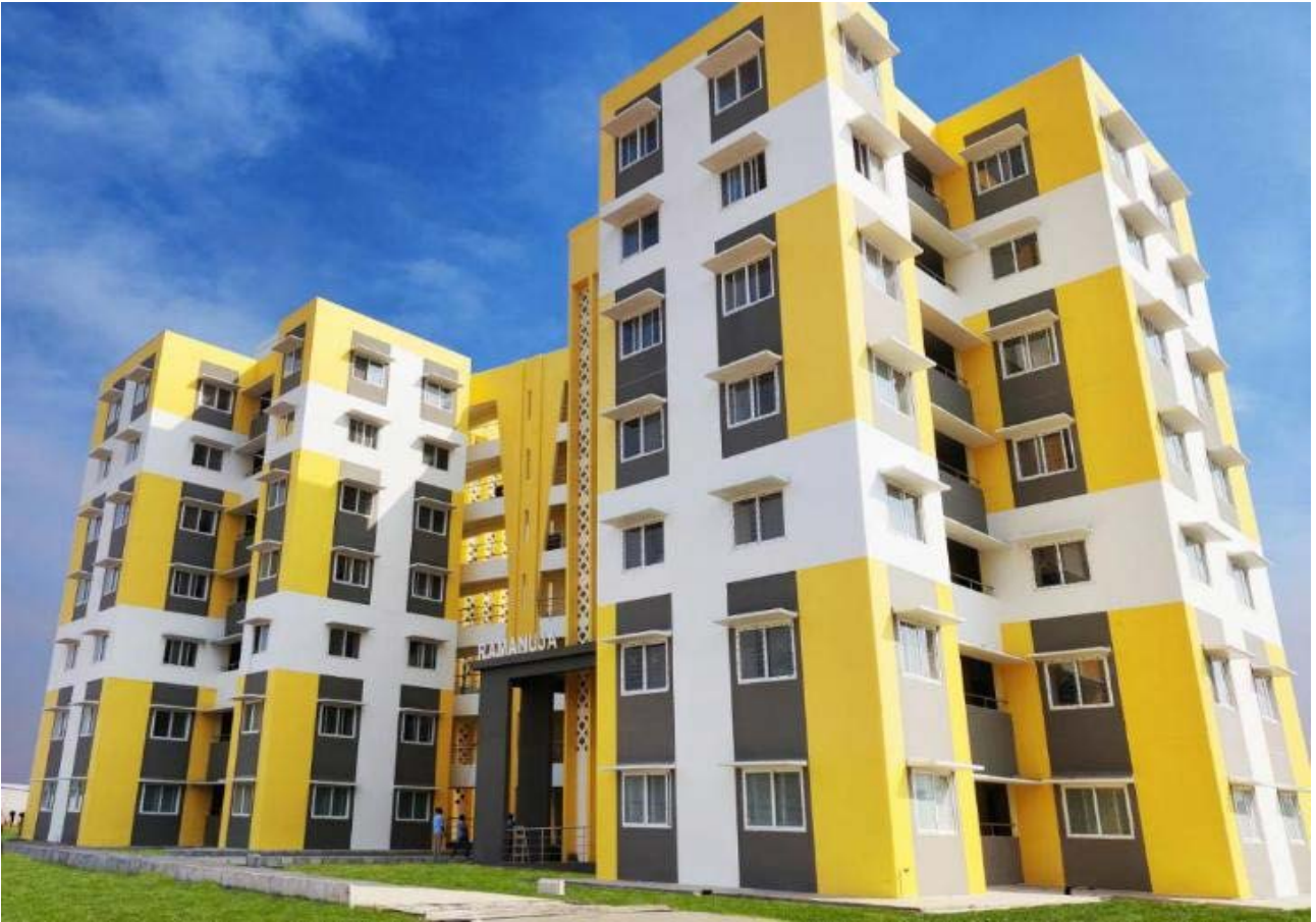
336 Nos Hostel Building (G+6) for Indian Institute of Technology at Hyderabad
