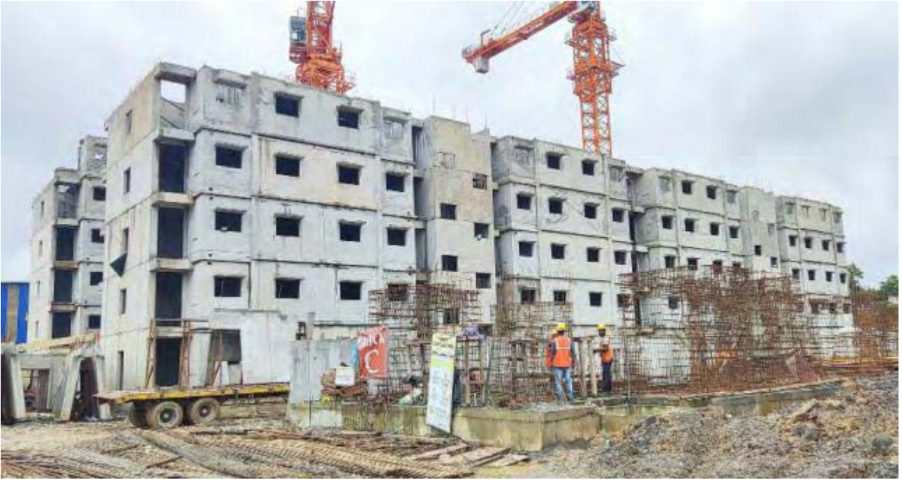
Light House project at Ranchi using 3D Volumetric Precast Construction
