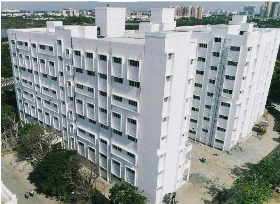
Hostel Beneficiaries and Associated Buildings (G+7) for National Institute of Empowerment of Persons with Multiple Disabilities at Muttukkadu – Chennai
