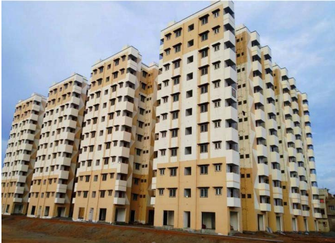
480 Multi Storeyed Tenements of Rehabilitation of NTO Scheme at Thiruvottriyur - Chennai
