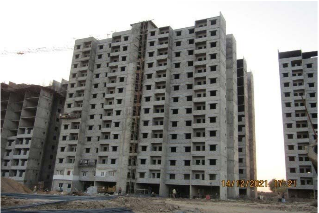
Light House Project at Rajkot under PMAY (U)
