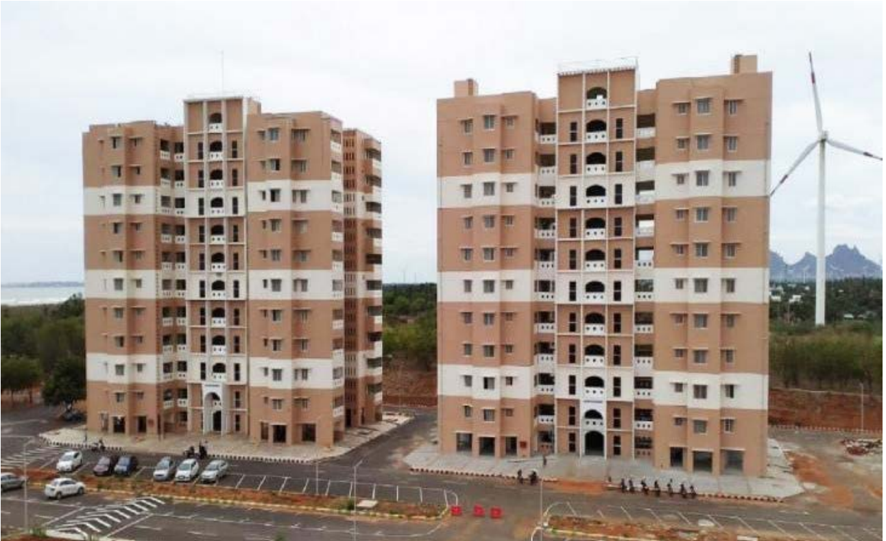
Executive Apartment Buildings (S+10) for Nuclear Power Corporation India Ltd
