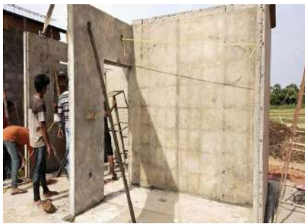
Wall Panels Erection
