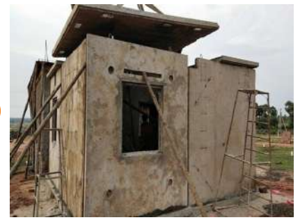
Roof Panel Erection
