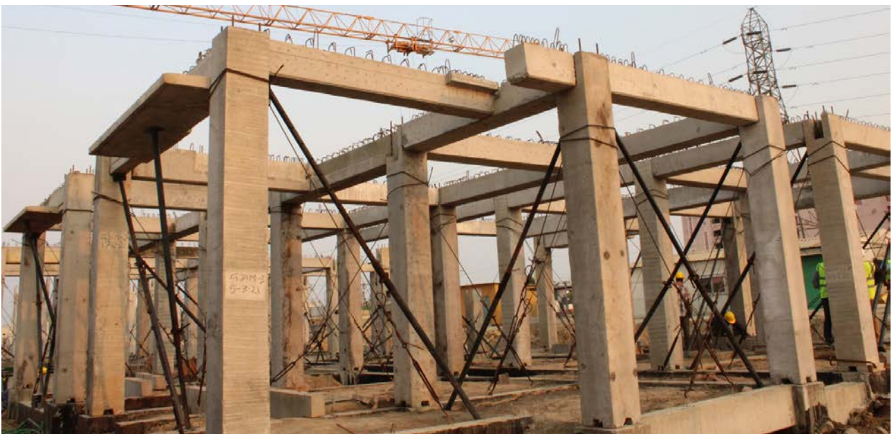
Placement of ground floor beam on columns
