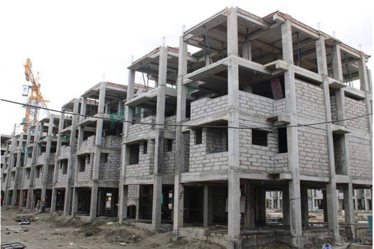
AAC block masonry work
