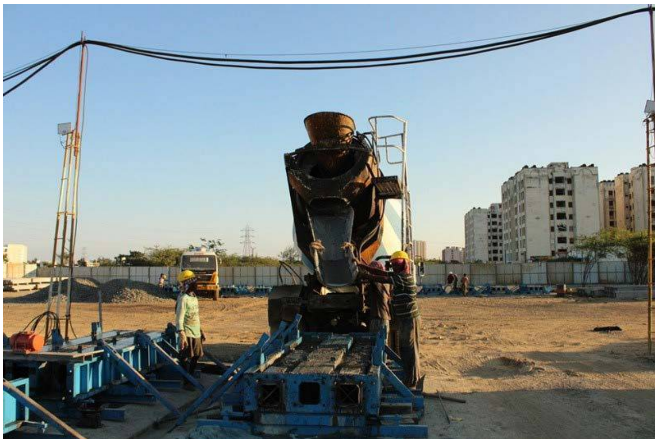
Manufacturing of column
