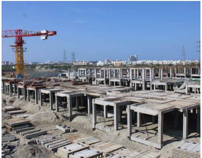
Erection of Floor/Slab
