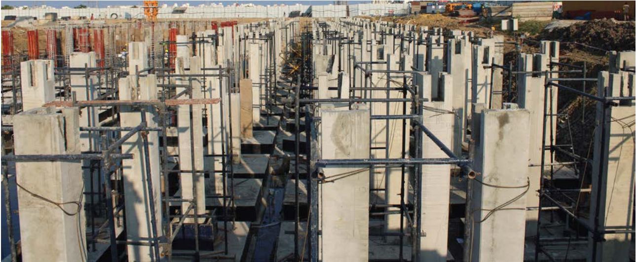
Erection of precast stem columns from footings
