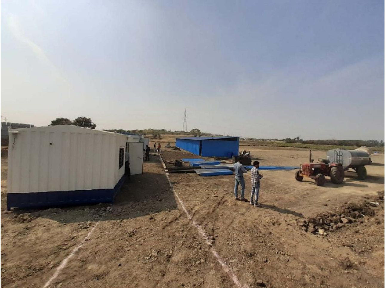
Layout marking for excavation
