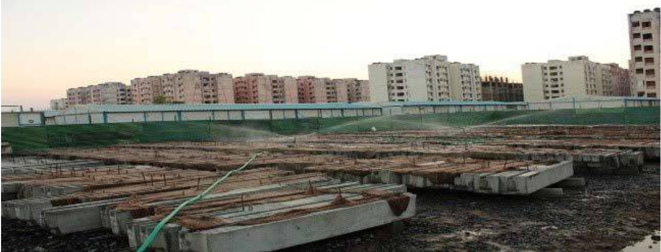
Precast RCC solid beams at site
