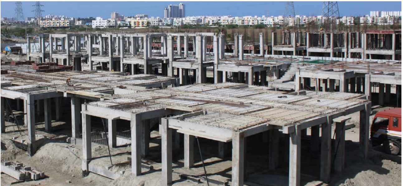
Reinforcement for screed concrete on partially precast slab
