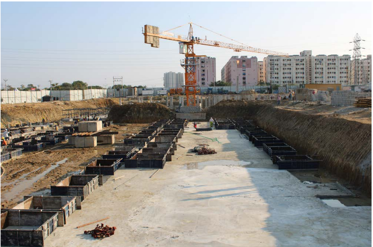
PCC and Shuttering for footings
