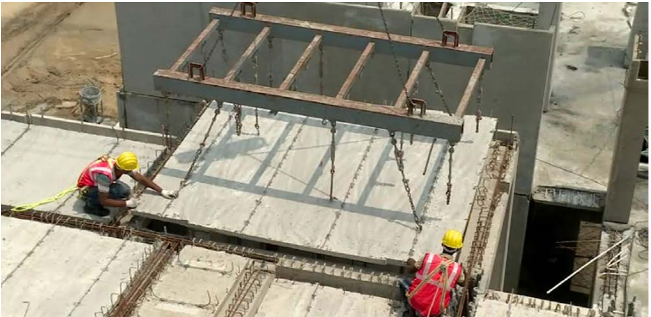
Placement of partially precast slab
