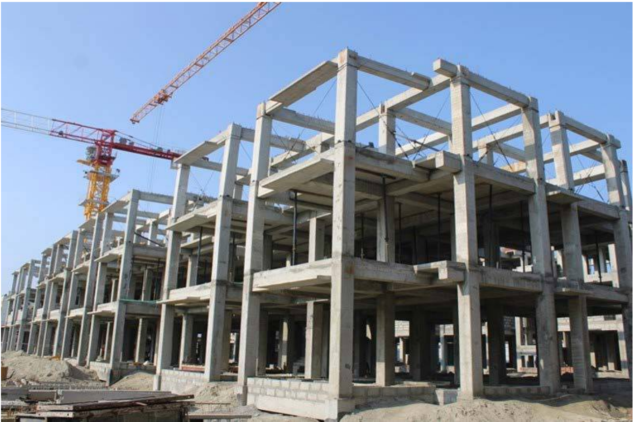
Erection of beams, columns and slab in upper floors
