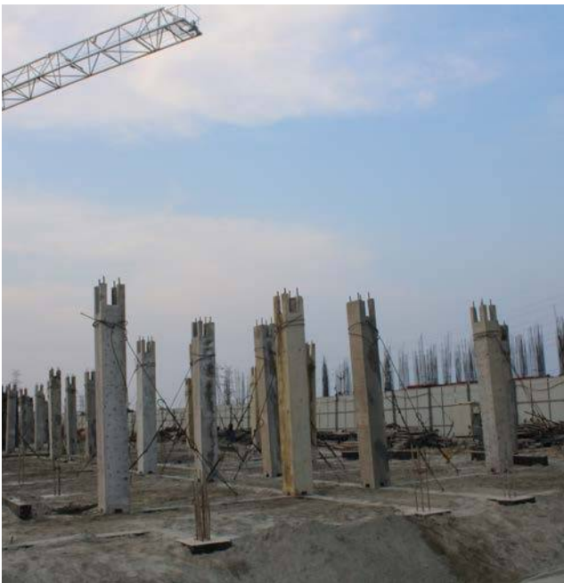
Assembly of precast columns and beam
