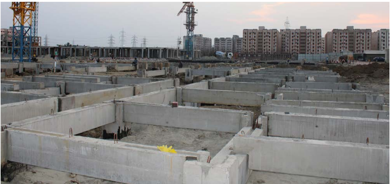
Precast plinth beam connection with stem columns
