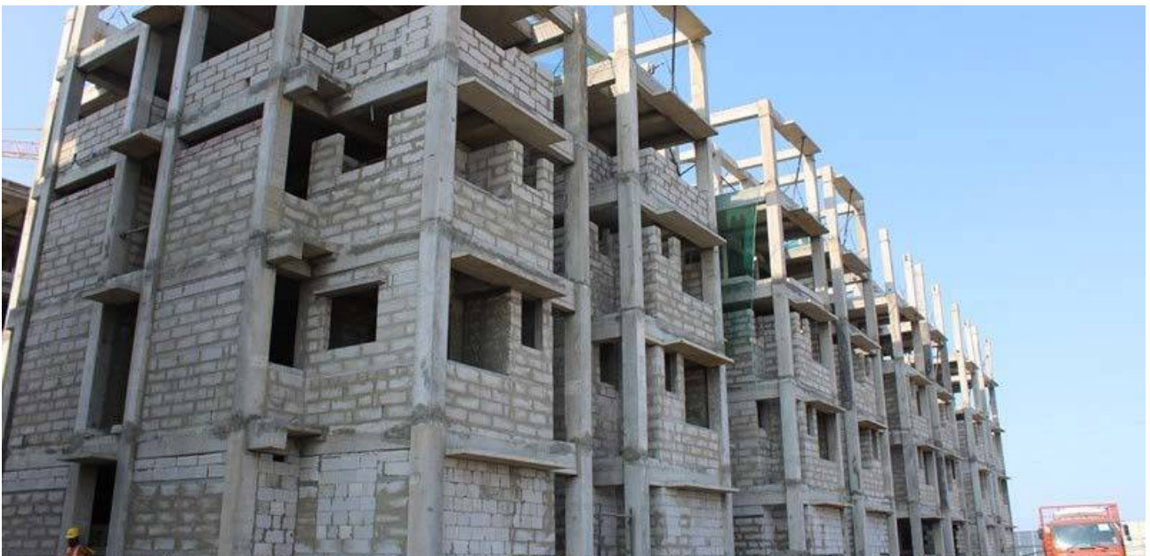
Erection of wall by Autoclaved Aerated Concrete (AAC) Blocks
