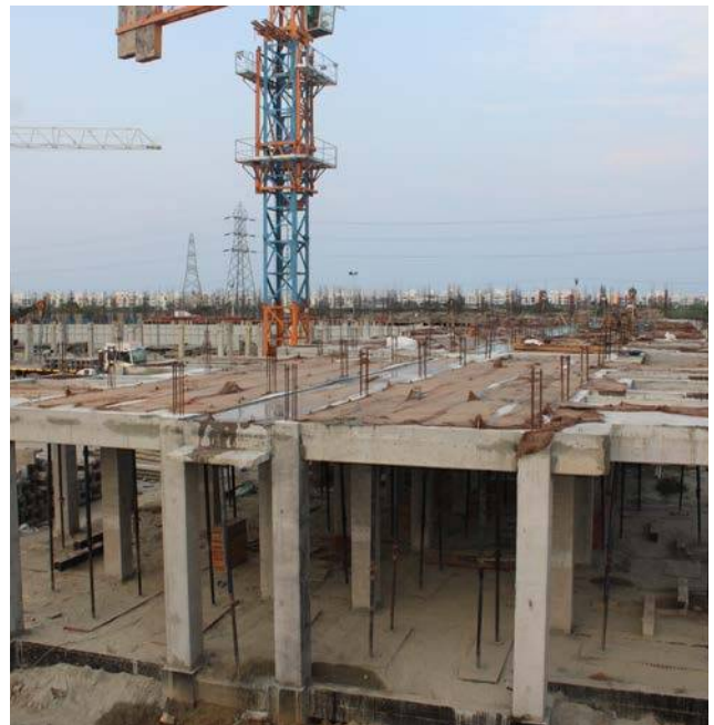
Assembly of precast columns and beam
