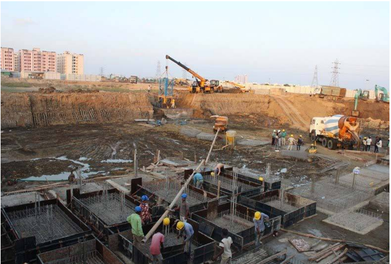
Shuttering and reinforcement work for footings
