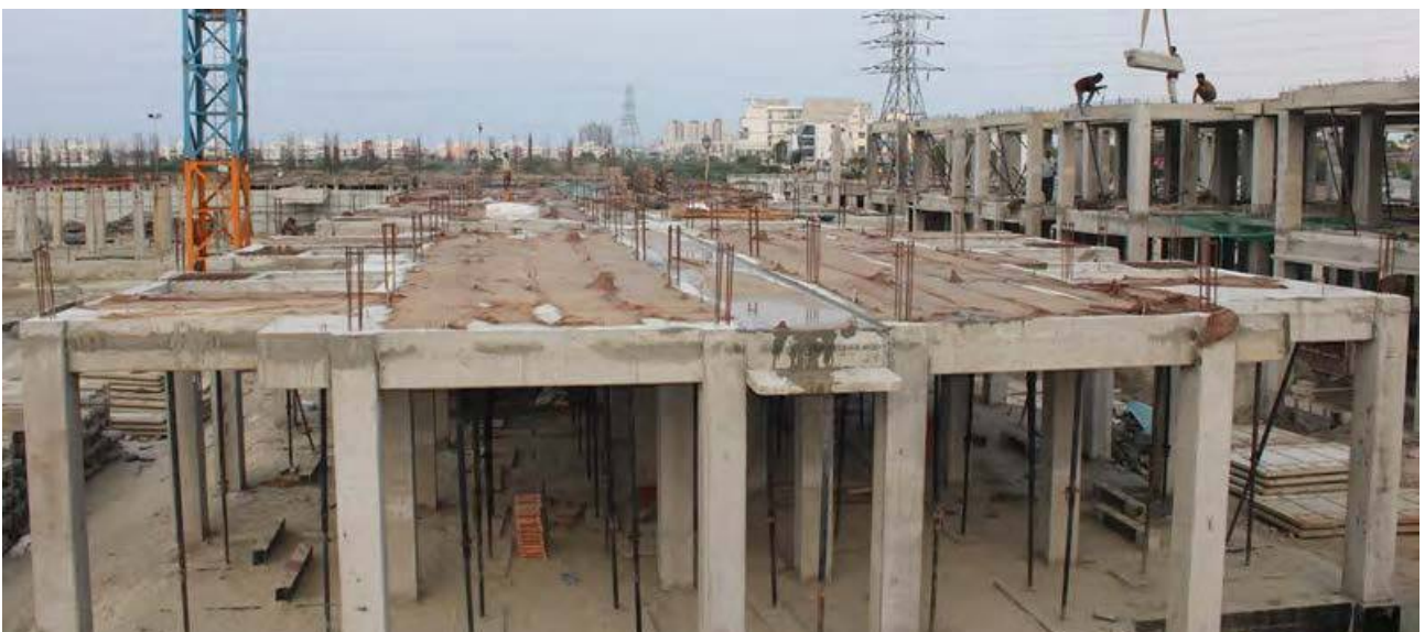
Monolithic RCC frame after screed concrete and wet jointing of beam, column and slab
