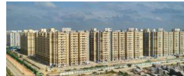
Construction of 1696 EWS & 280 Cat. II houses and Construction of 2561 EWS & 419 Cat. II houses by using Prefab Technology at Narela, New Delhi by B.G.Shirke
