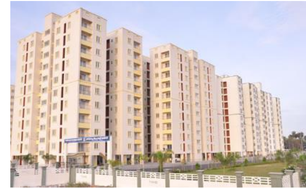
Construction of 1500 (G+10) Multi Storey Housing Project with Prefab Technology at Sholinganallur for Tamilnadu Housing Board, Chennai by B.G.Shirke
