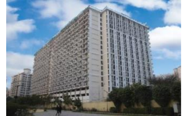
Omkar Pawai, Transit Camp, Mumbai, Total Built up Area : 3.5 lac sqft G+7, 5 bldgs/ 205 sqft (1 BHK ) 1,700 units by HIL Limited
