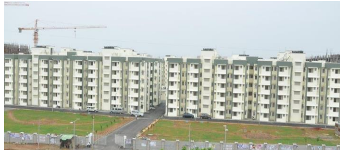
Light House Project (1152 DUs, G+5) in Chennai by B.G.Shirke
