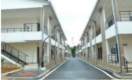
Houses for Orissa Power Generation Corporation, Jharsuguda, Orissa by Everest Industries Ltd.
