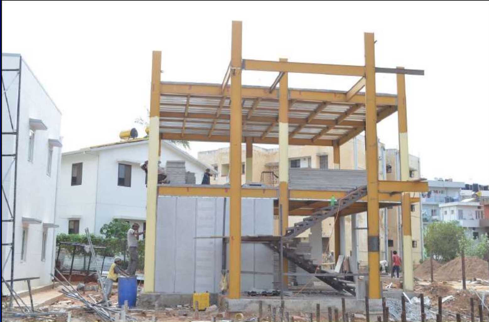
Steel skeleton with Aerocon panel infills
