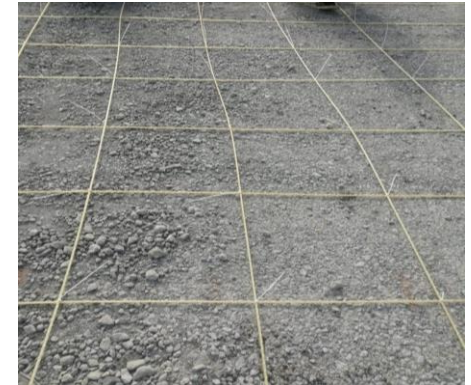
Road Construction Aurangabad
