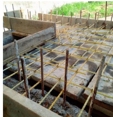
Water Sump - Chennai
