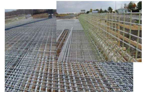
Bridge Decks & Barriers
