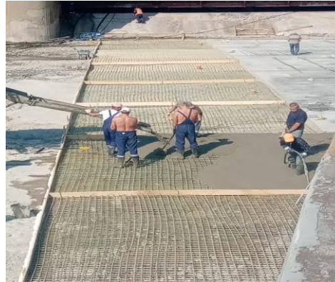
Dam Construction, Russia
