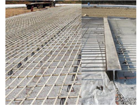
Highway Construction USA - 2008
