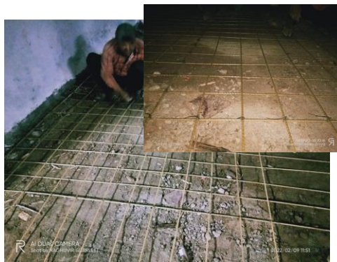
Commercial Building Basement Trimix Raghuvir Builders, Surat
