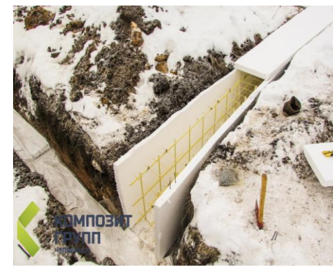
Strip foundation - Russia
