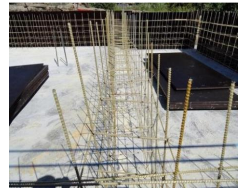
Retaining Walls - Chennai
