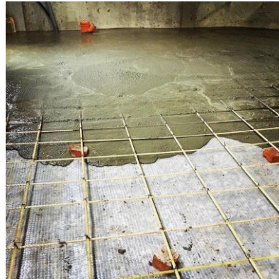
Basement PCC – Shaligram Builders, Ahmedabad
