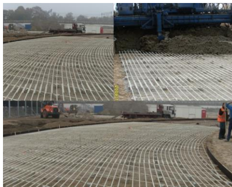
Eindhoven airport Runway CRCP - Netherlands 2009
