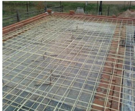
Residential Building Slab - Chennai
