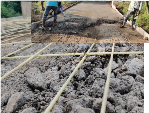
Road Construction – Forest Department, Gir, Gujarat
