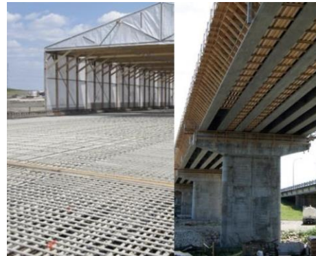
Brandon Bridge - Canada 2010
