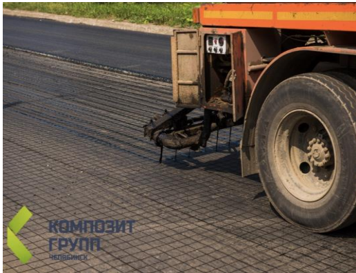
Road paving with composite mesh Russia
