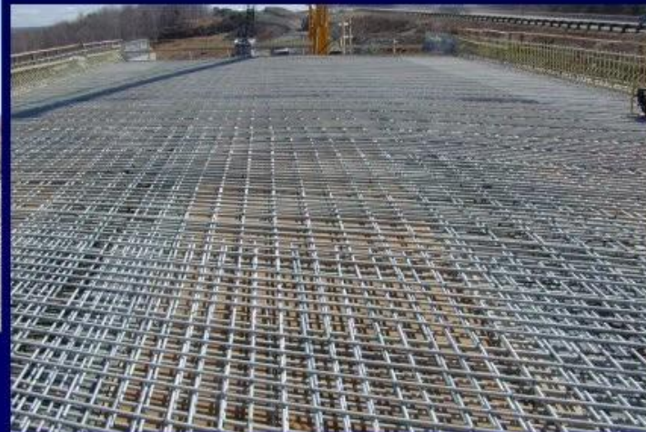
Placement of Glass FRP Bars
