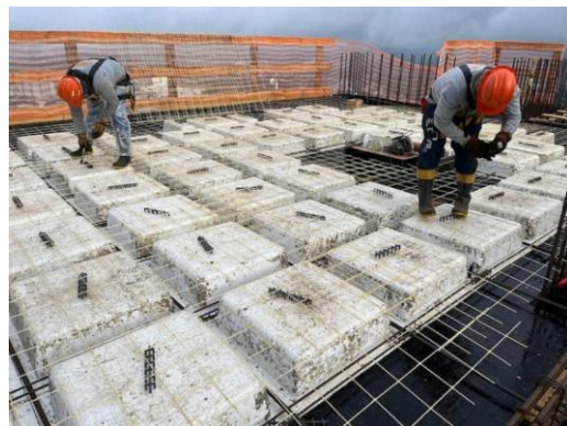
Void Slabs - Residential Building Brazil
