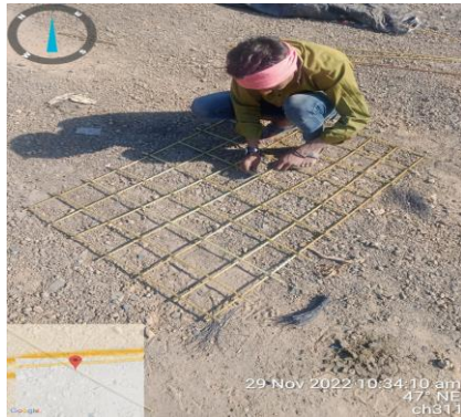
Drain Precast Slabs – NHA1 Project, L&T, Gadhidham
