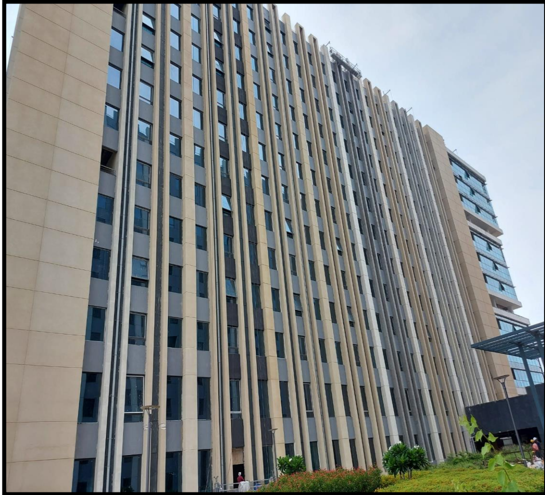
STAGE-3- EIFS INSTALLATION COMPLETED
