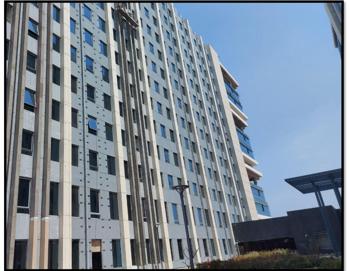
STAGE-2- ALUMINIUM PROFILE BRACKET INSTALLATION
