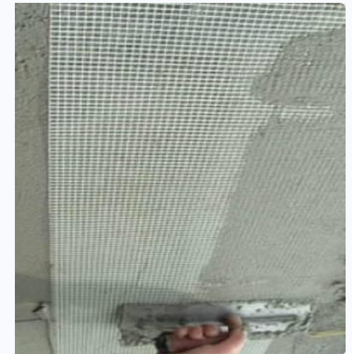
Non-shrink grout with glass-fiber mesh
