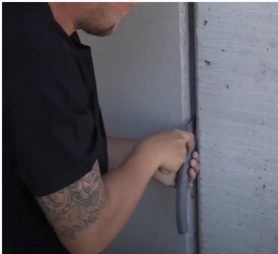
Backer rod installation
