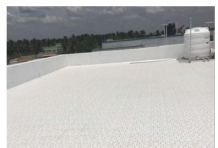
Reflecting. Reflects the sun rays away from the building
