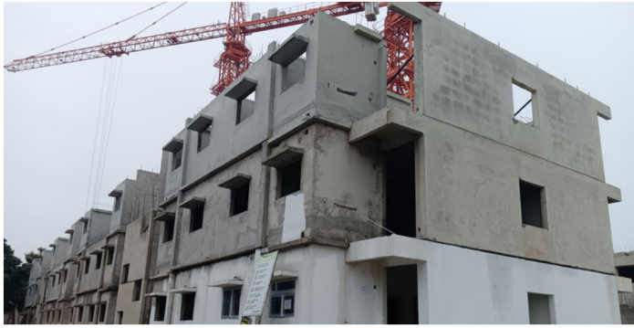
Photo: Building 1 - Pod & Panel Erection, Internal Wall Grouting, Putty at the LHP Ranchi Site
