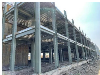
PEB & DECK SLAB STRUCTURE
