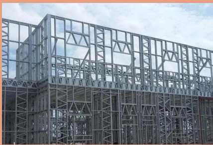
Light Gauge Steel Structure System
