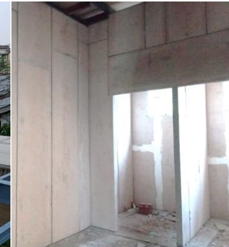
Flyash EPS Cement Sandwich Panels with steel structure
