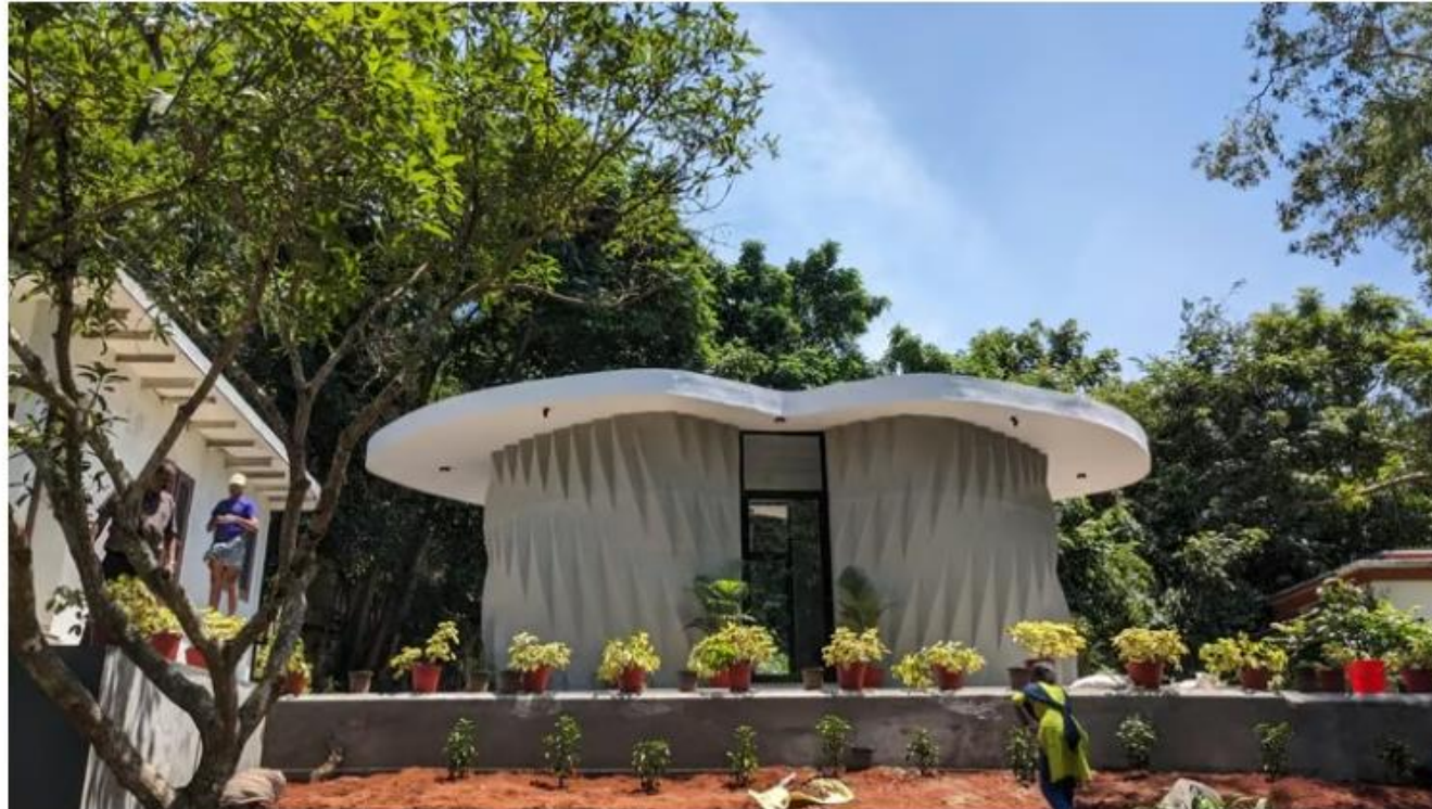
'AMAZE-28' that was built using 3D printing technology
