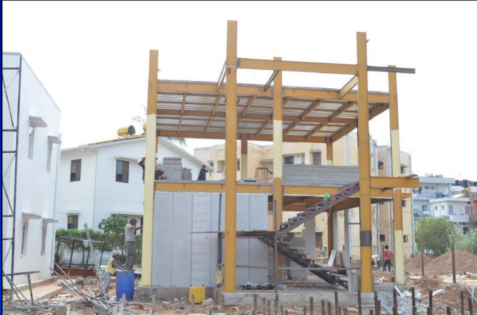
Steel skeleton with Aerocon panel infills
