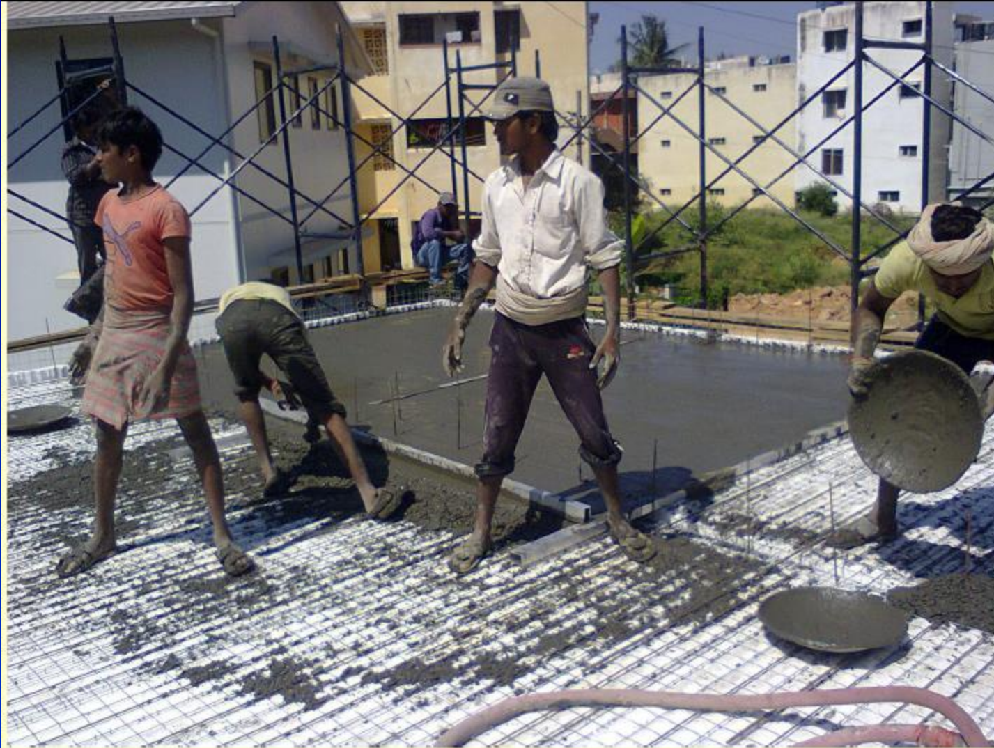
Concreting of floor
