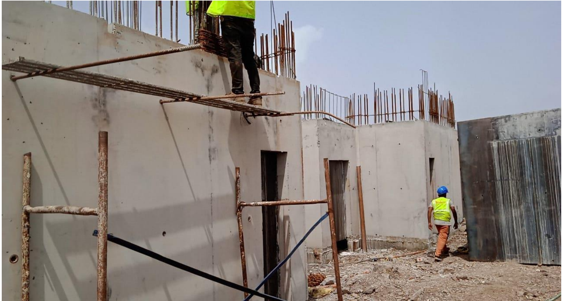
Shear Wall after removal of Tunnelform
