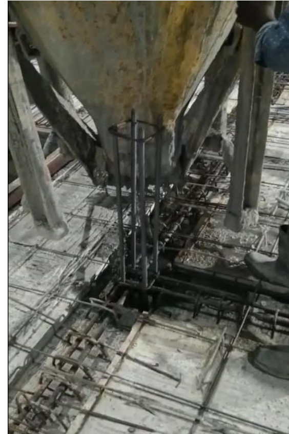
Beam - column - slab wet jointing
