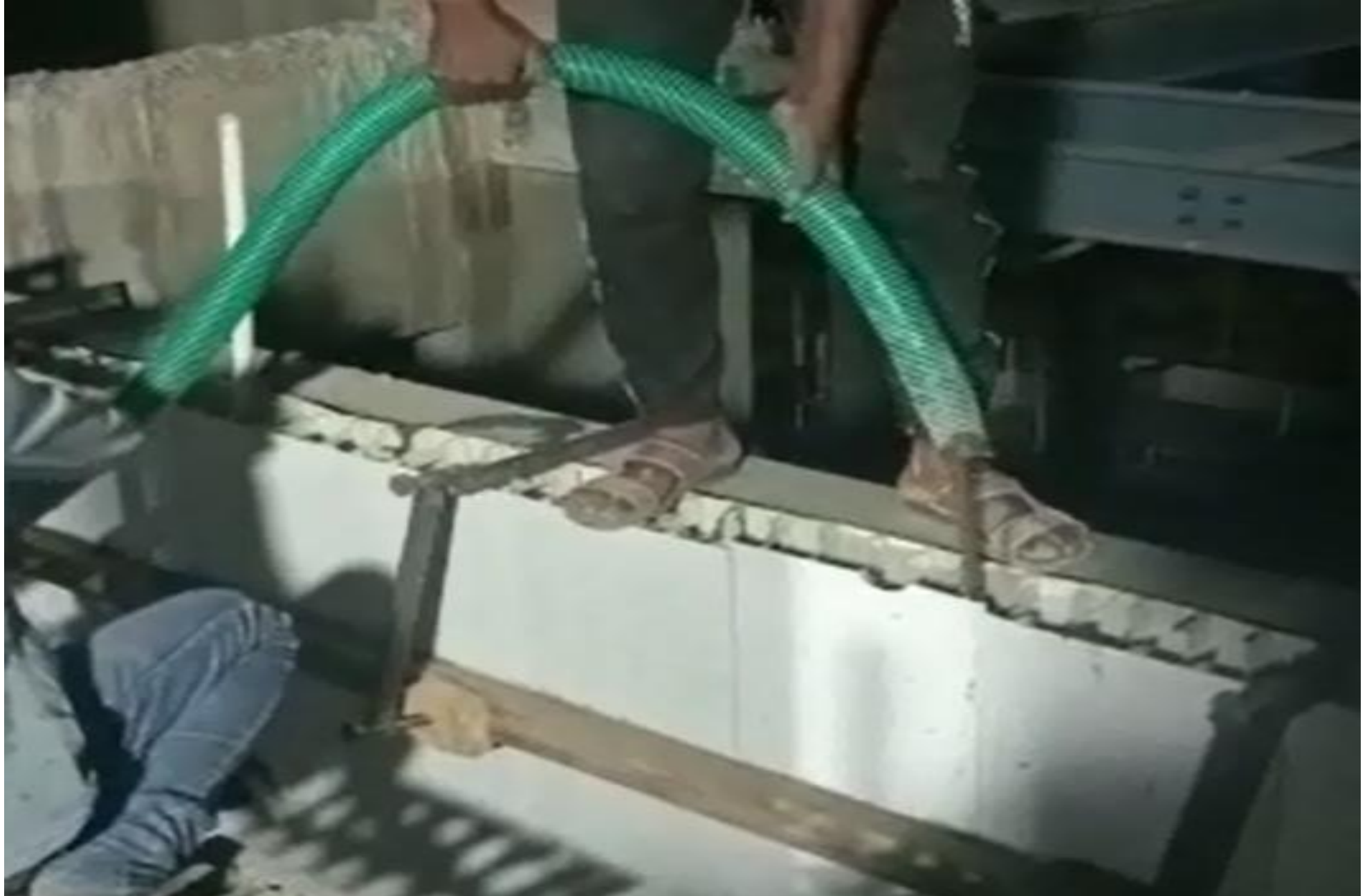
Concreting in Wall
