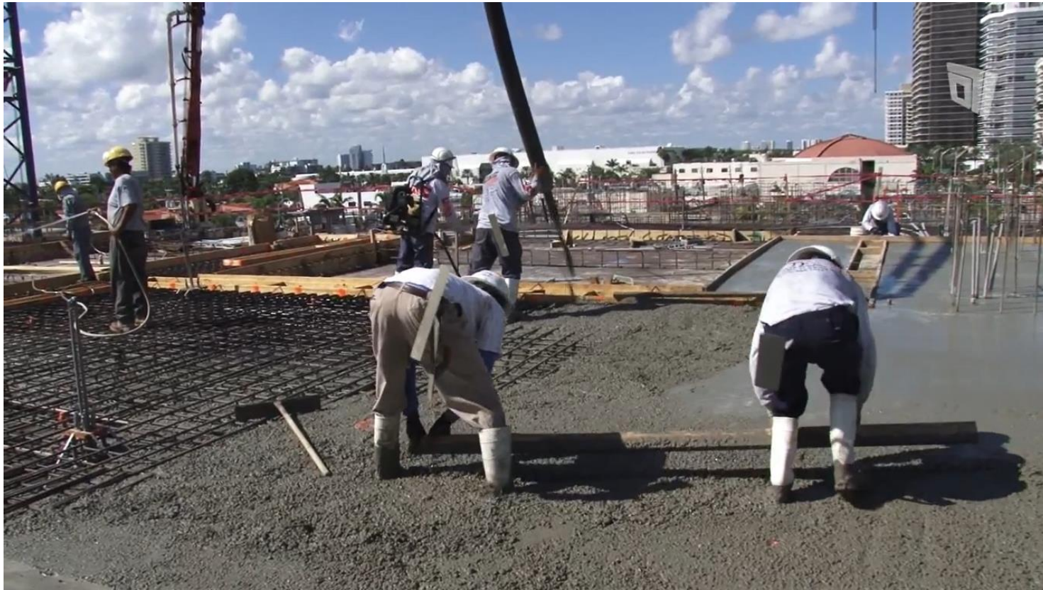
Placement and leveling of concrete
