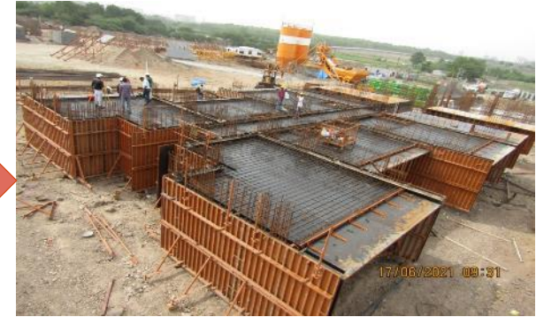
Assembly of Formwork
