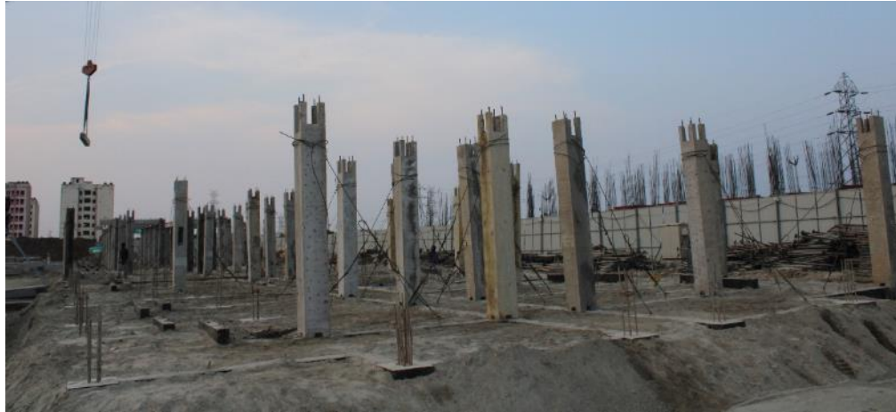
Erected Precast columns with notches and dowels over plinth beam
