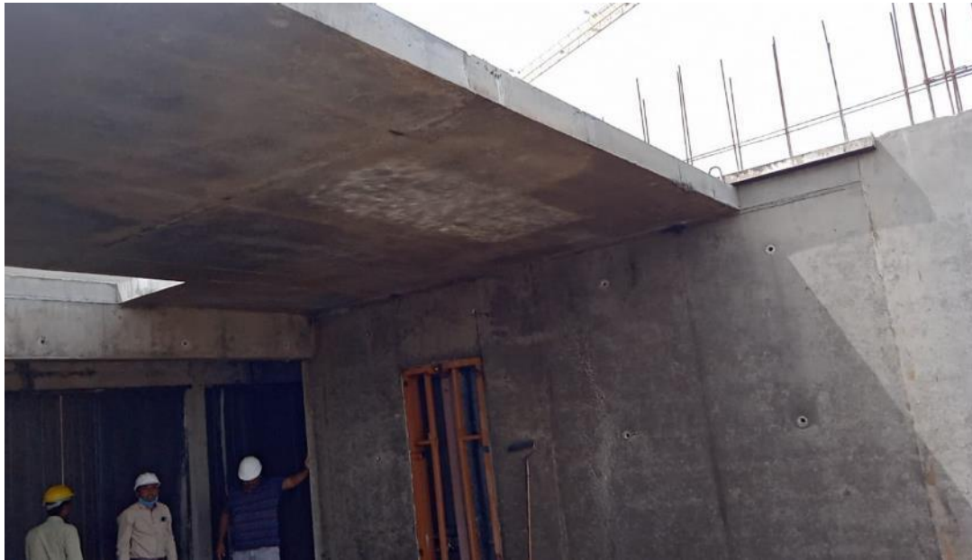
Shear Wall and Slab after removal of Tunnelform
