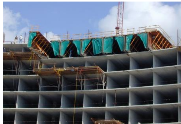
Structure after removal of formwork - Shear Wall Construction
