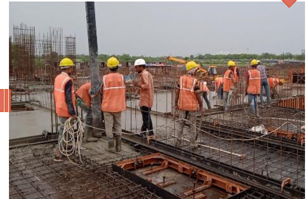
Concreting after Placing formwork
