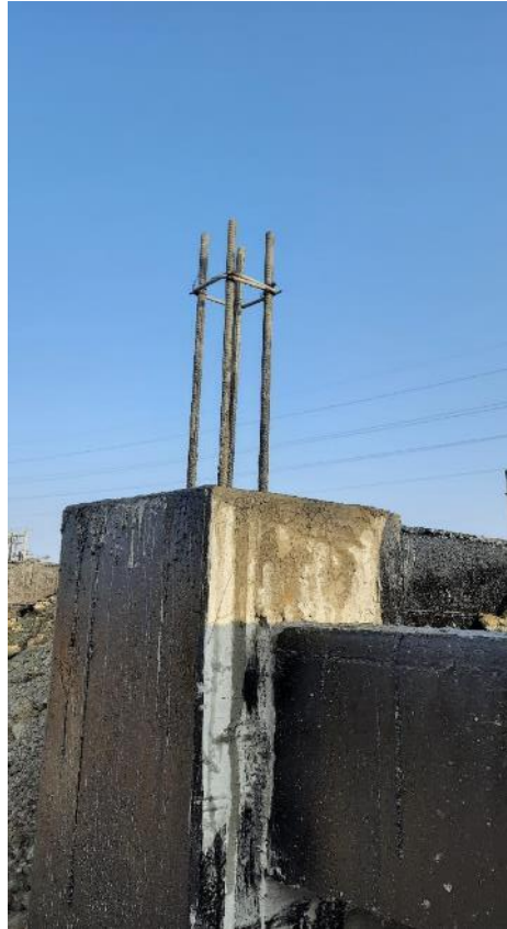
Grouting of beam - column joint
