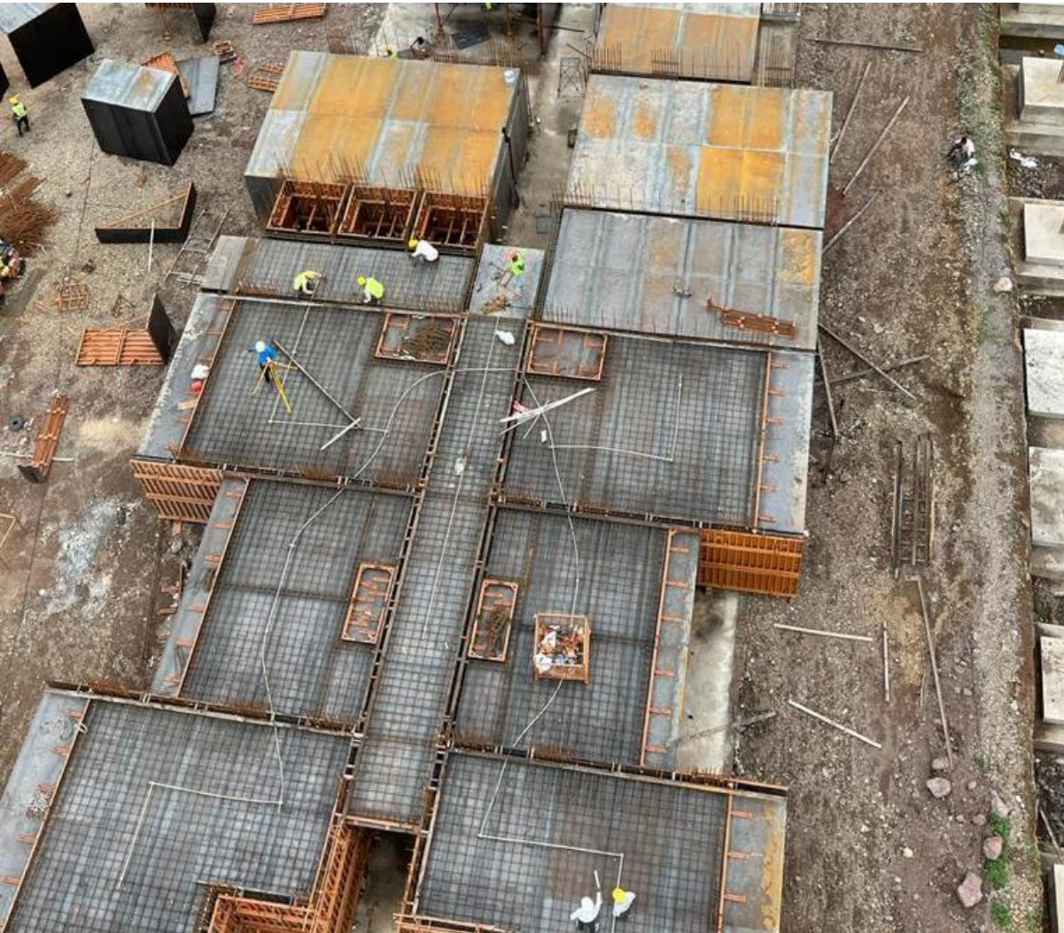
Typical Reinforcement at Slab level
