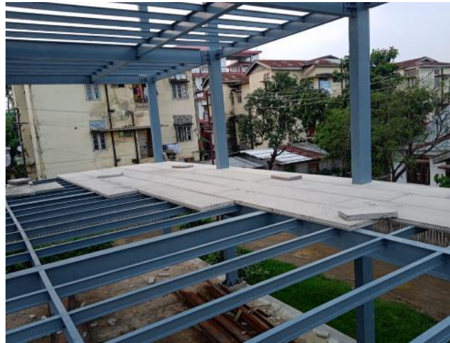
Flyash EPS Cement Sandwich Panels with steel structure
