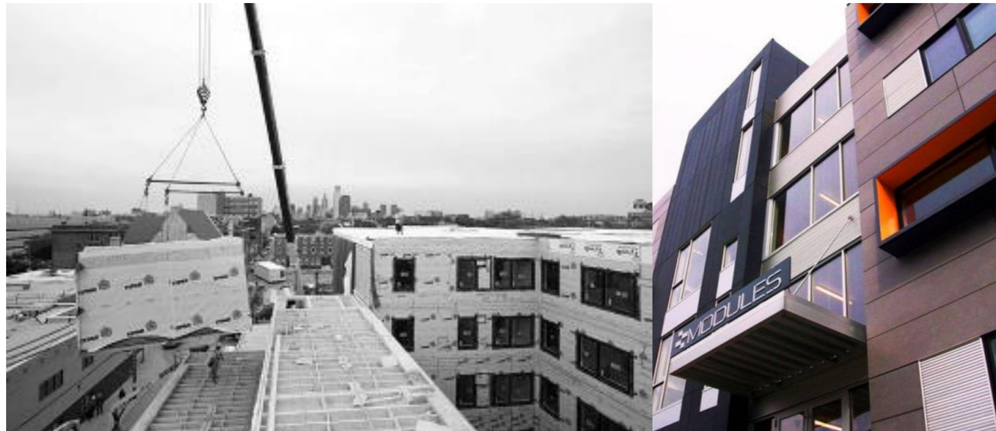
The Modules, Philadelphia, Constructed in 2010 using Wooden based modules, approx. 80,000 and 160 bed.
