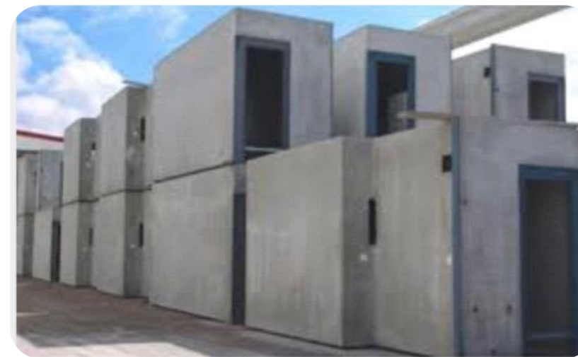
Casting of Modules
