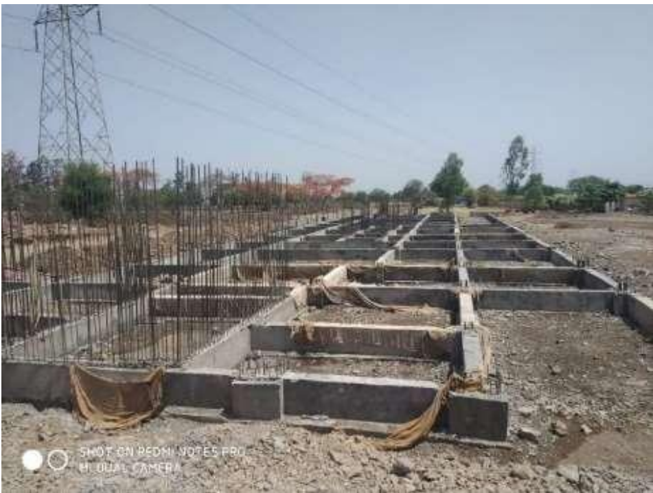
RCC COLUMN UP TO PLINTH LEVEL
