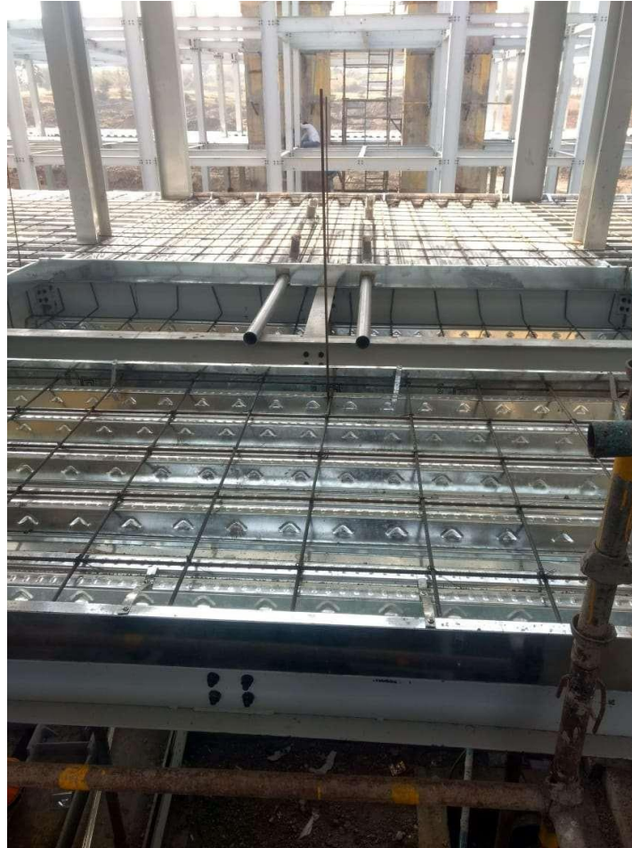
Services & Reinforcement Laying
