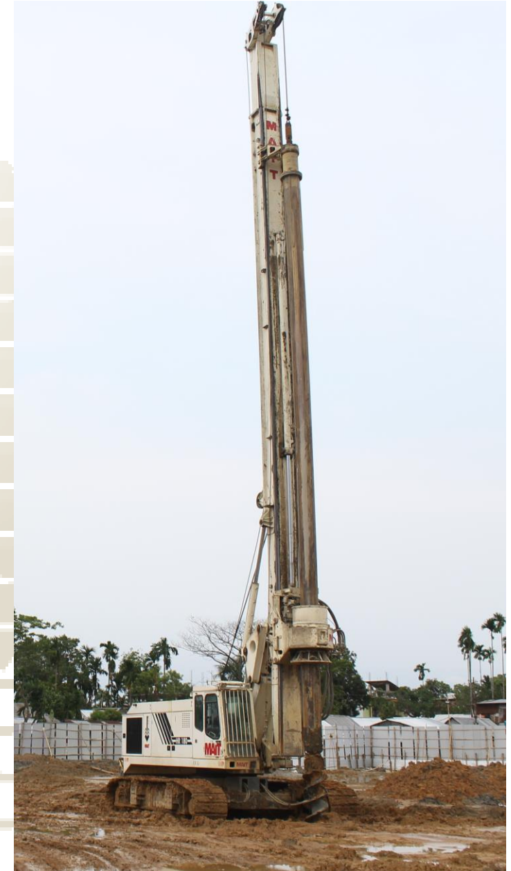
Excavation & Pile Head Breaking
