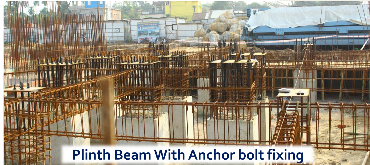
Raft Steel Binding
