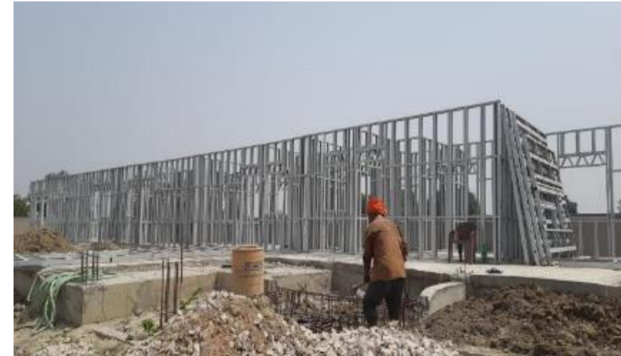
Light Gauge Steel Frame structure with cement fiber board
