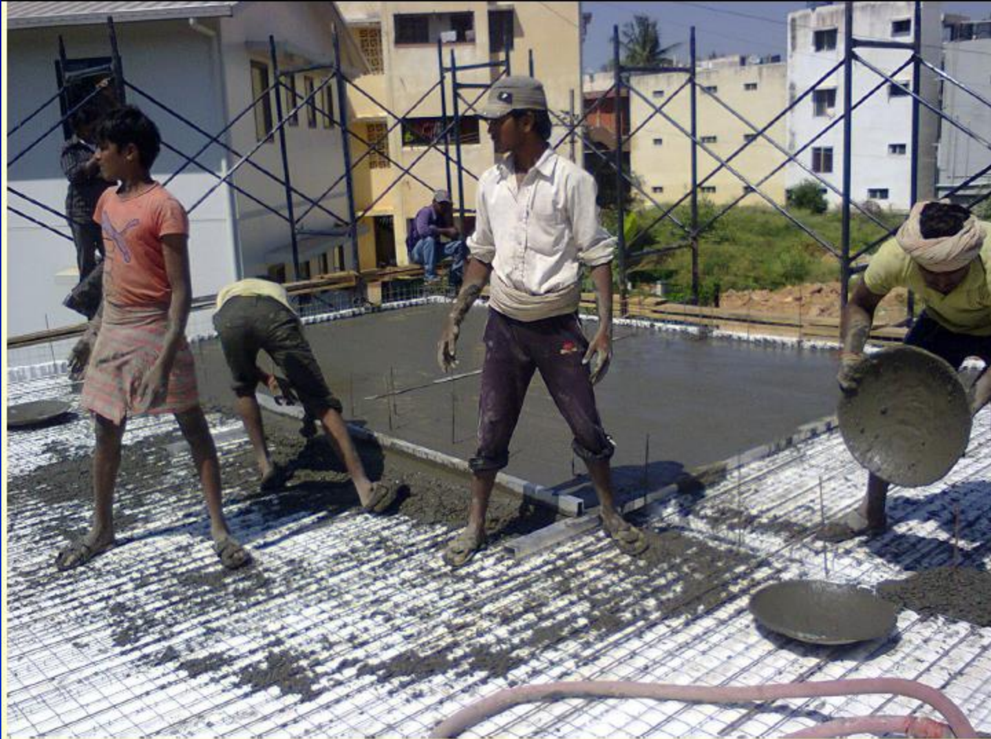
Concreting of floor
