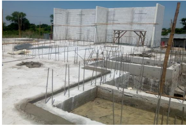
EPS core panel using Quikbuild Panels
