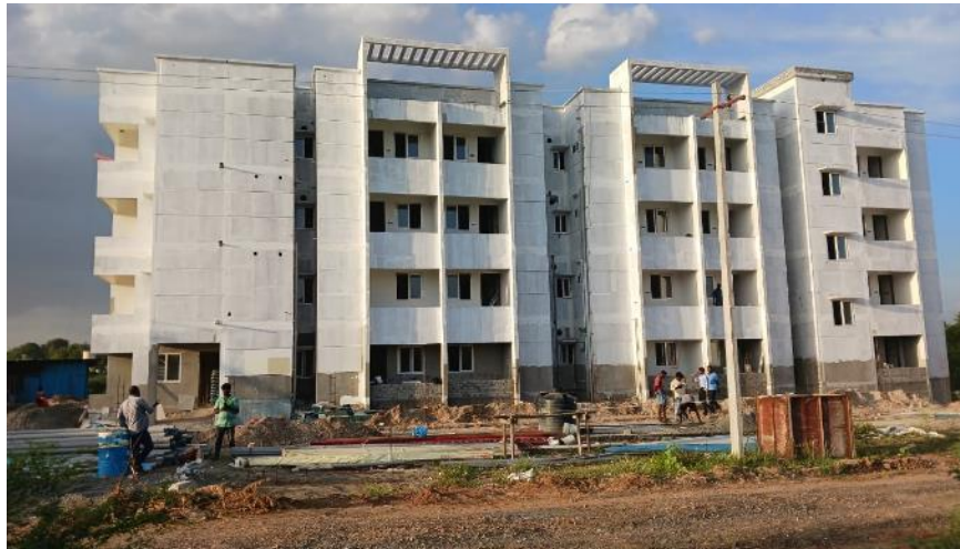
Precast Concrete Construction System
