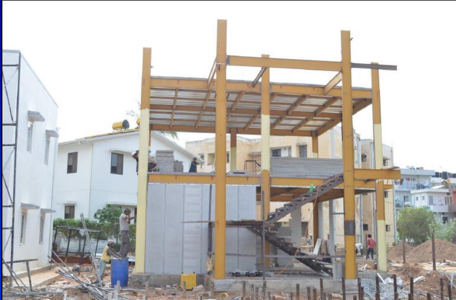
Steel skeleton with Aerocon panel infills
