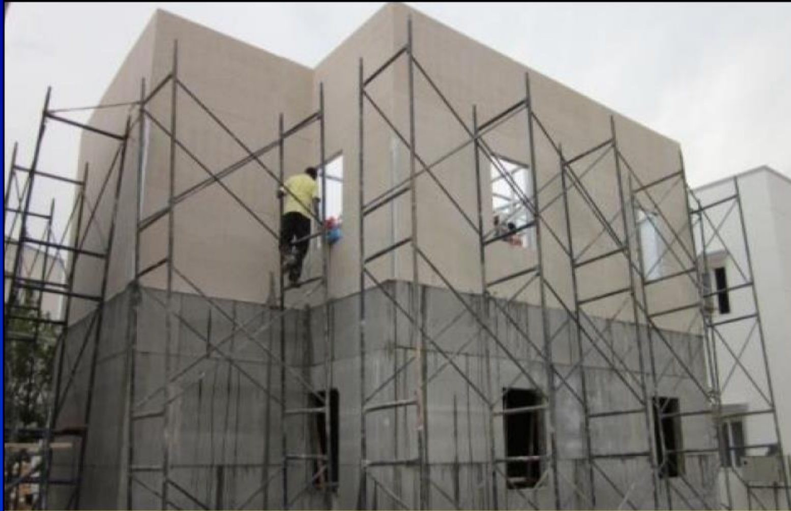
Composite construction - In-situ concrete floor and roof
