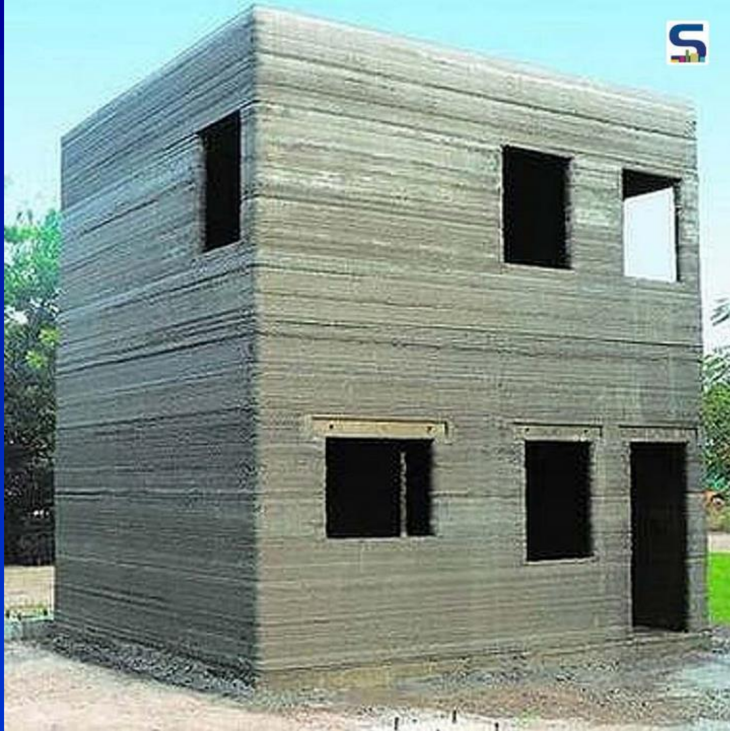
3D Printed House at Kanchipuram by L & T
